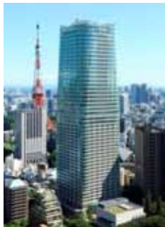
ARK Hills Sengokuyama Mori Tower
