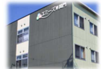
Izuhakone Railway Lines Combined facility for short-stay and day services Emies Higashimakado
