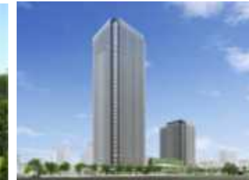
Hotel in the "Global Gate" in Nagoya(Opening)
