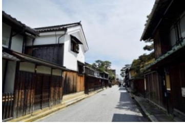
Hachiman Preservation District for Groups of Historic Buildings
