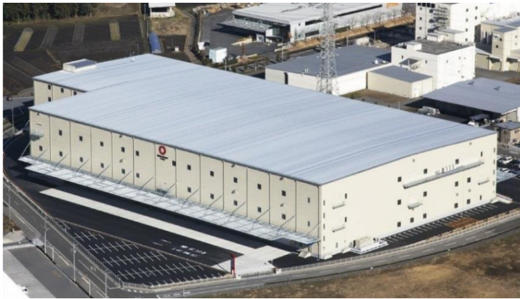
(Property Number) LB-054 D Project Kaminokawa
