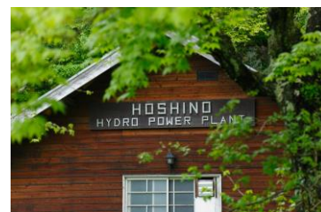
Hydro power plant helps power the heat pump
