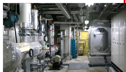
Heat pump system uses ground-source thermal and hot spring water outflow as thermal source for air conditioning and hot water supply
