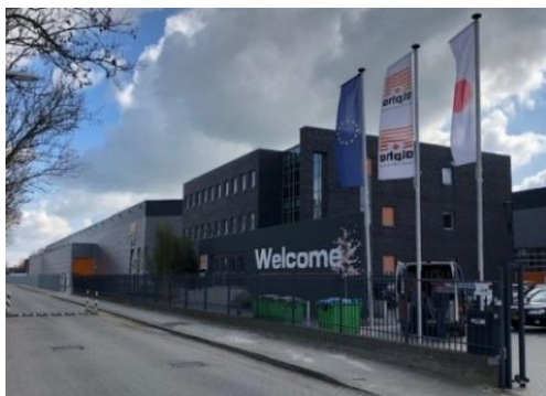
New office building
