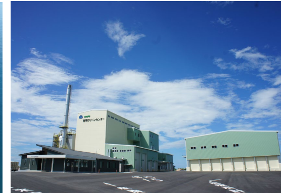
(Working title) Construction work of Ariake Clean Center (Kumamoto pref.)
