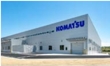
Seal ring factory at Himi Plant
