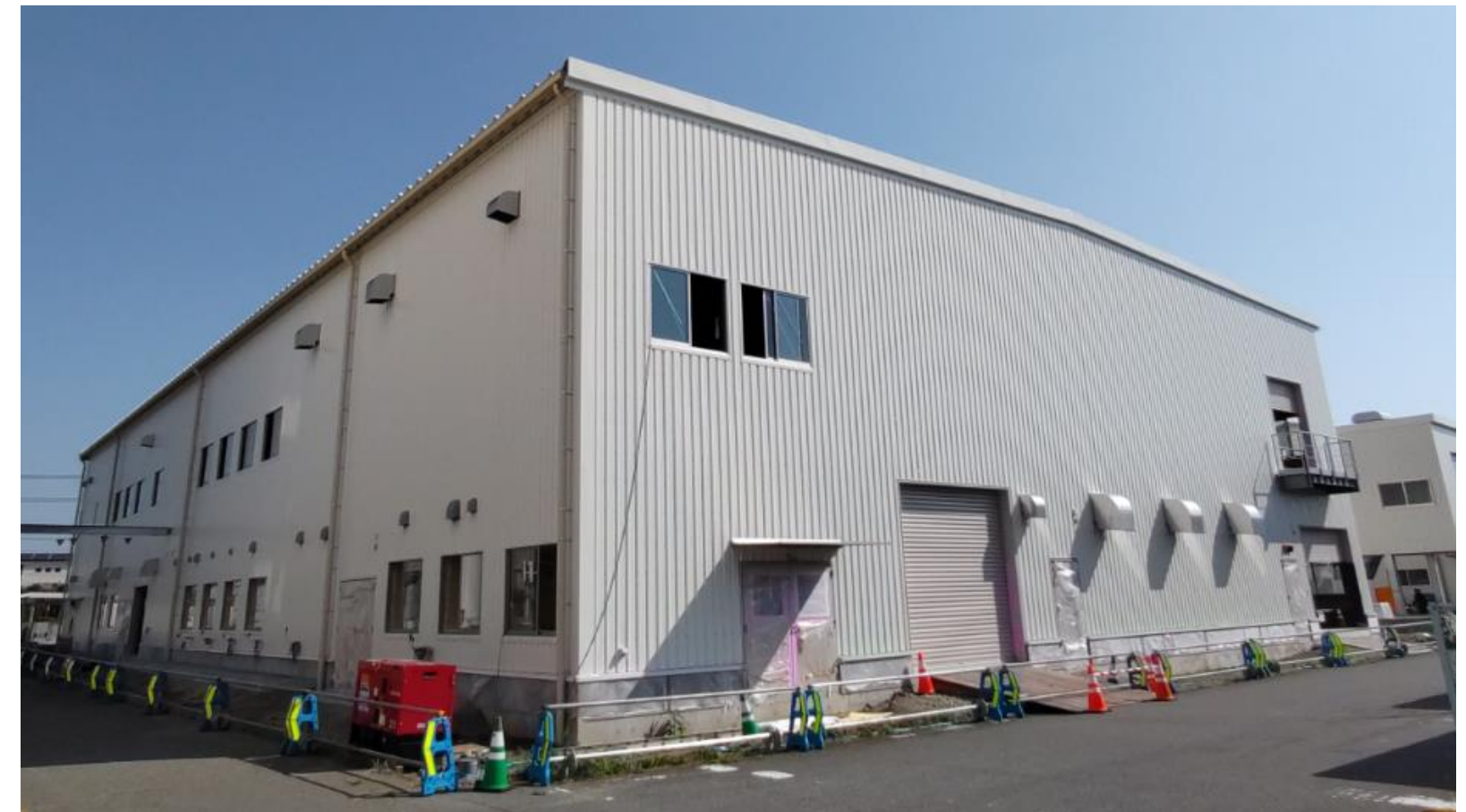
Building for new production line in Chigasaki City
