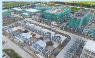
Construction status as of last year
