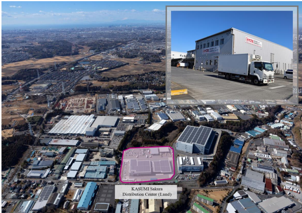
KASUMI Sakura Distribution Center (Land) Photo of the property
