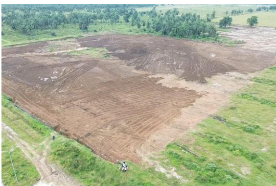
Construction site of plant
