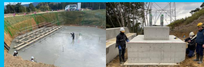
Concrete Placement (Dec. 2024)
