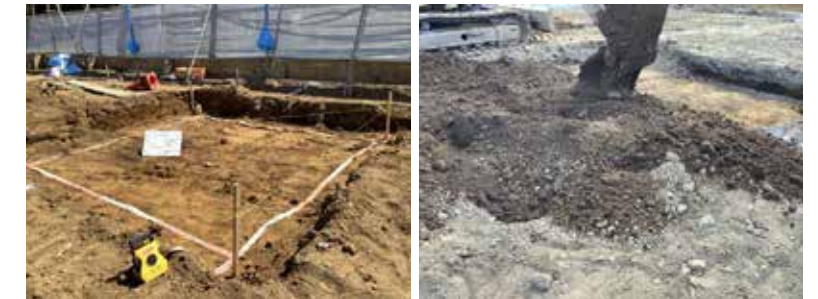
Left: Identification of the contaminated area Right: Replacement with healthy soil
