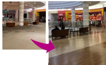
Floor replacement work
