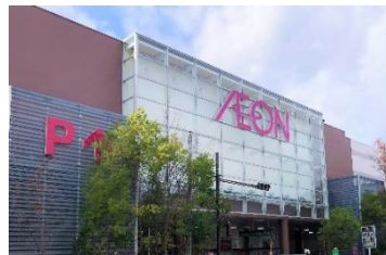
Exterior wall painting
