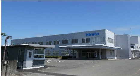
Exterior View of Shichijo Plant No.2
