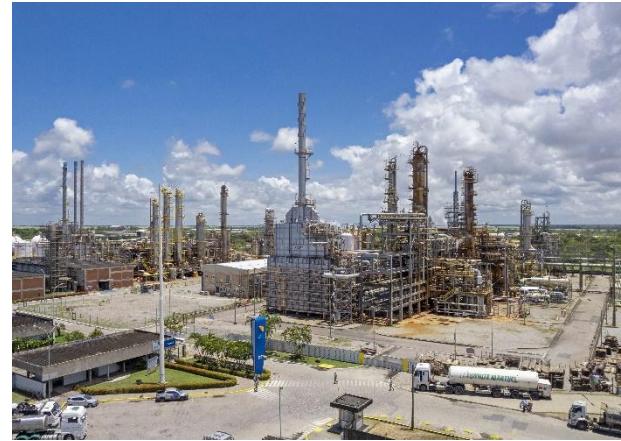
Braskem VCM plant (Photo courtesy of Braskem)
