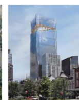
Torch Tower (Building B)
