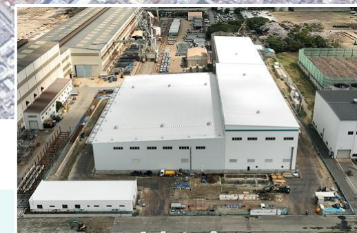
Ichihara Sorting Center under construction (April 2026)
