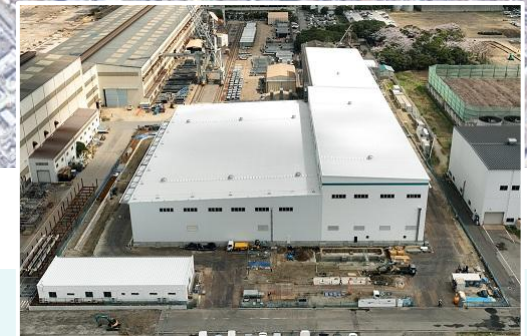
Ichihara Sorting Center under construction (April 2026)
