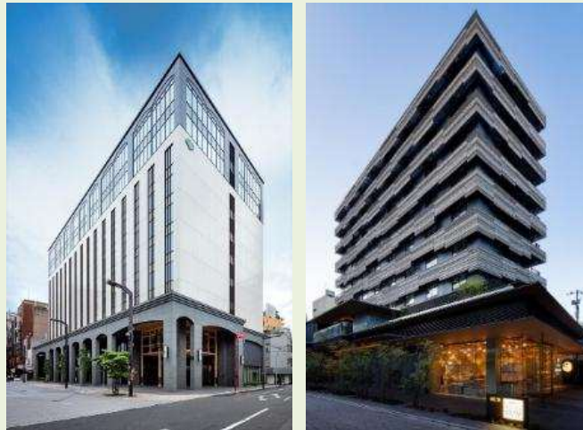
Asakusa Rokku Shochiku Building (Asakusa View Hotel ANNEX ROKKU) Kyoto Shochiku Sakaiza Building(Tokyu Stay Kyoto Sakaiza) Hakata ST Building(Hakata Excel Hotel Tokyu), etc.
